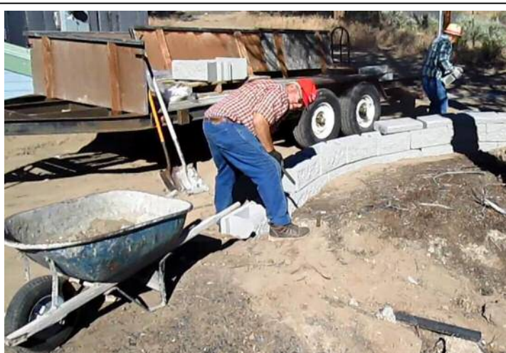
Wayne & Marie building the retaining wall in front of office.
